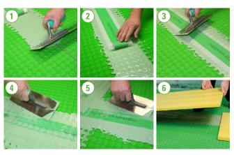
6 After laying, protect the surface of the membrane immediately from frequent foot traffic and direct abrasion using wooden planks or panelling.
