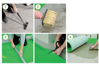
If the installation is external, leave a 5 mm joint between one sheet and the next.
