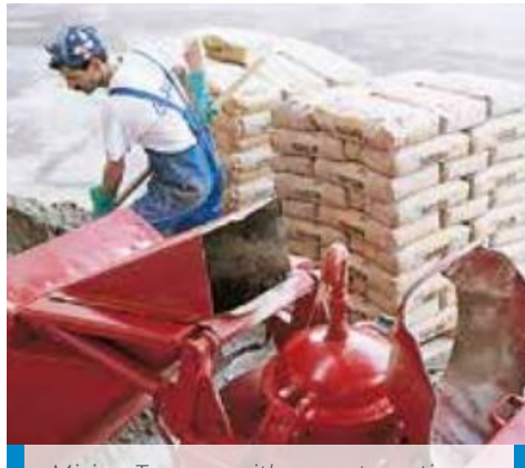
Mixing Topcem with an automatic pumping unit
