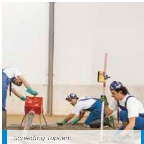
Mixing Topcem with an automatic pumping unit
