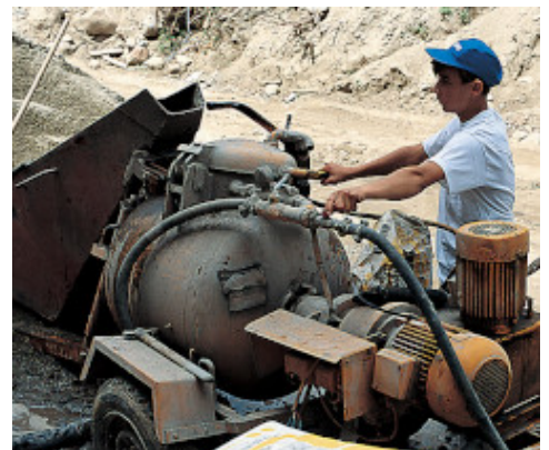
Mixing Mapecem with an automatic pumping unit
