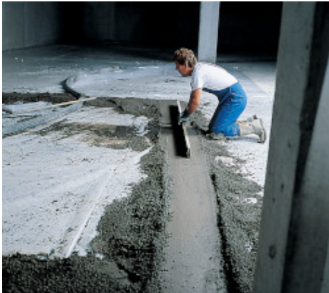
Preparing a levelling strip
