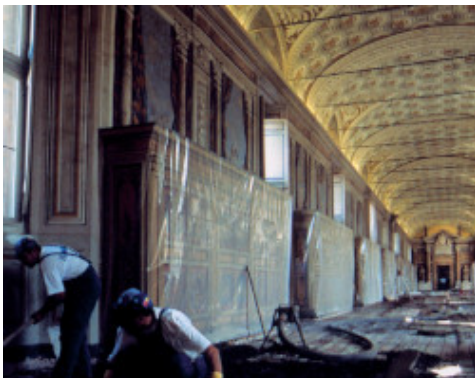
Laying and smoothing of the Mapecem screed - Sistine Halls - Vatican City
