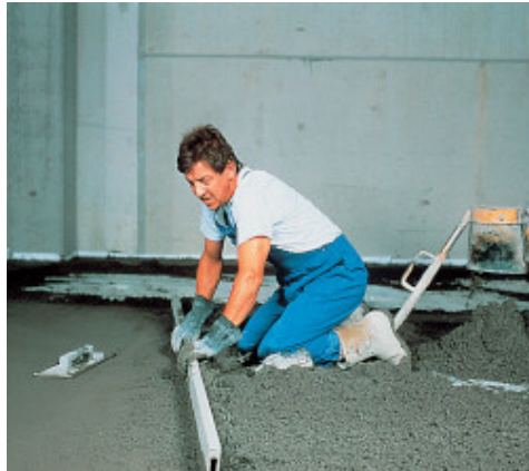
Using the straight-edge
