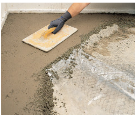
Covering pipes with Mapecem and reinforcement netting
