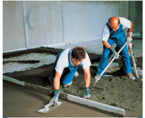
Fast repair of a screed in a supermarket
